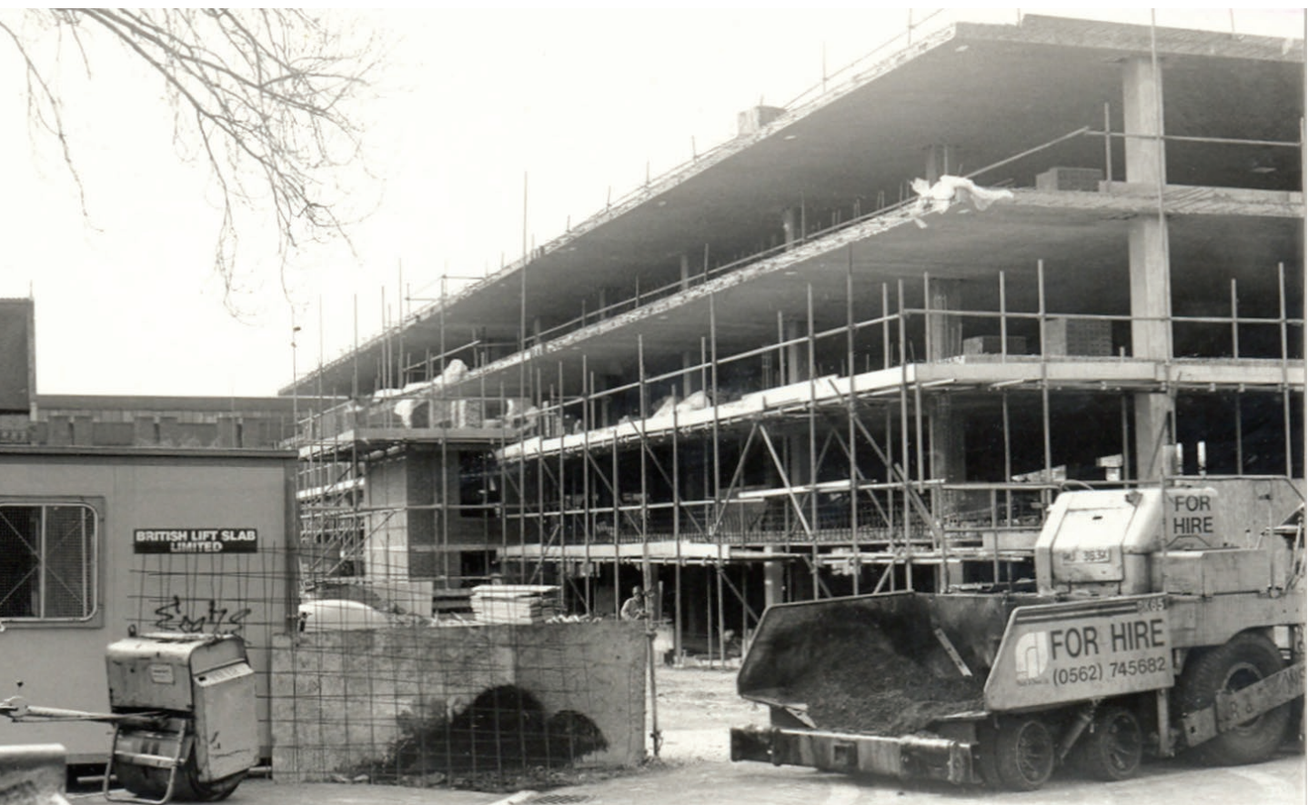
St. Martin's Gate Multi-storey car park under construction
