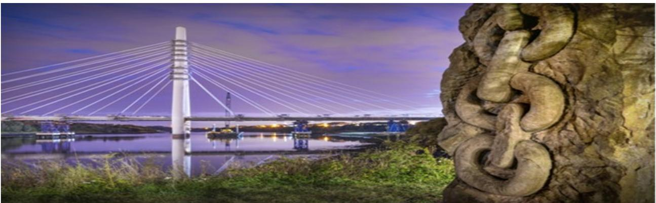
The new road bridge is a two-span cable-stayed bridge with an A-frame pylon rising to 105m (344ft) crossing the River Wear between Castletown on the north to Pallion on the south bank.
