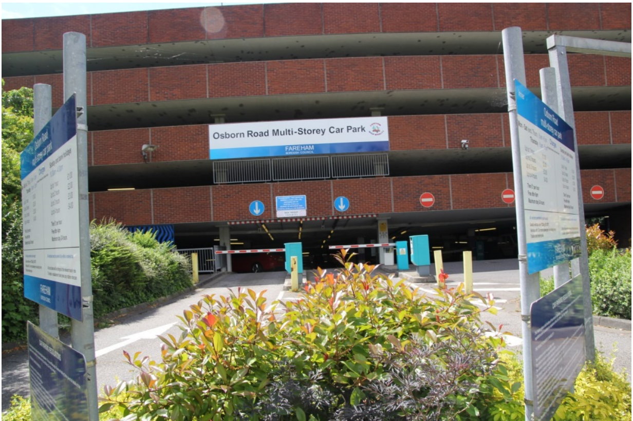
Osborn Road Multi-Story Car Park
