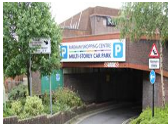
Fareham Shopping Centre Multi-storey
