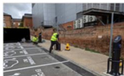
EV Points being installed in Avlesbury
